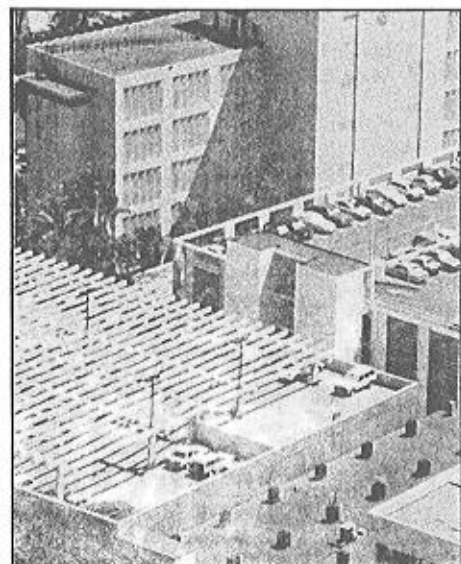
Trellis-work to soften visual impact of rooftop parking
