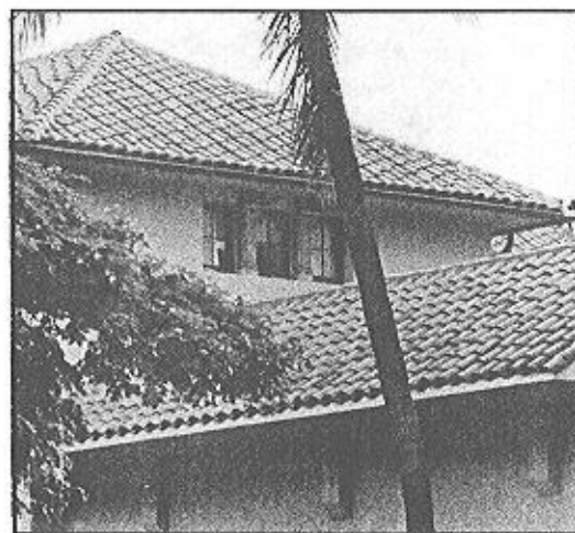
Honolulu Hale, an example of the Spanish-Mediterranean style using reddish, straight barrel mission tiles.
