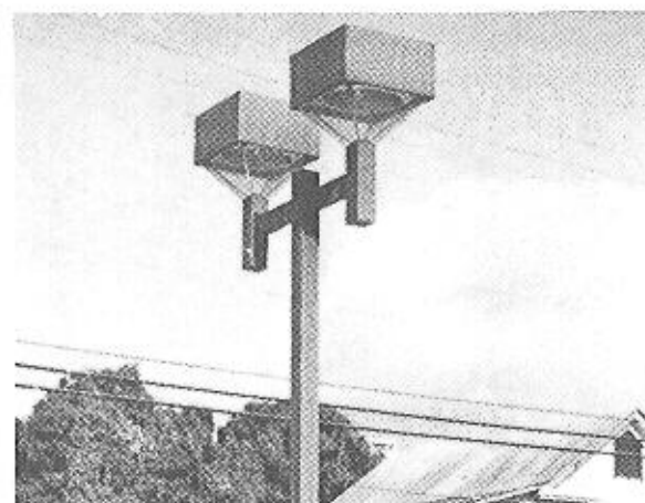
Acceptable shielded parking lot light fixture.
